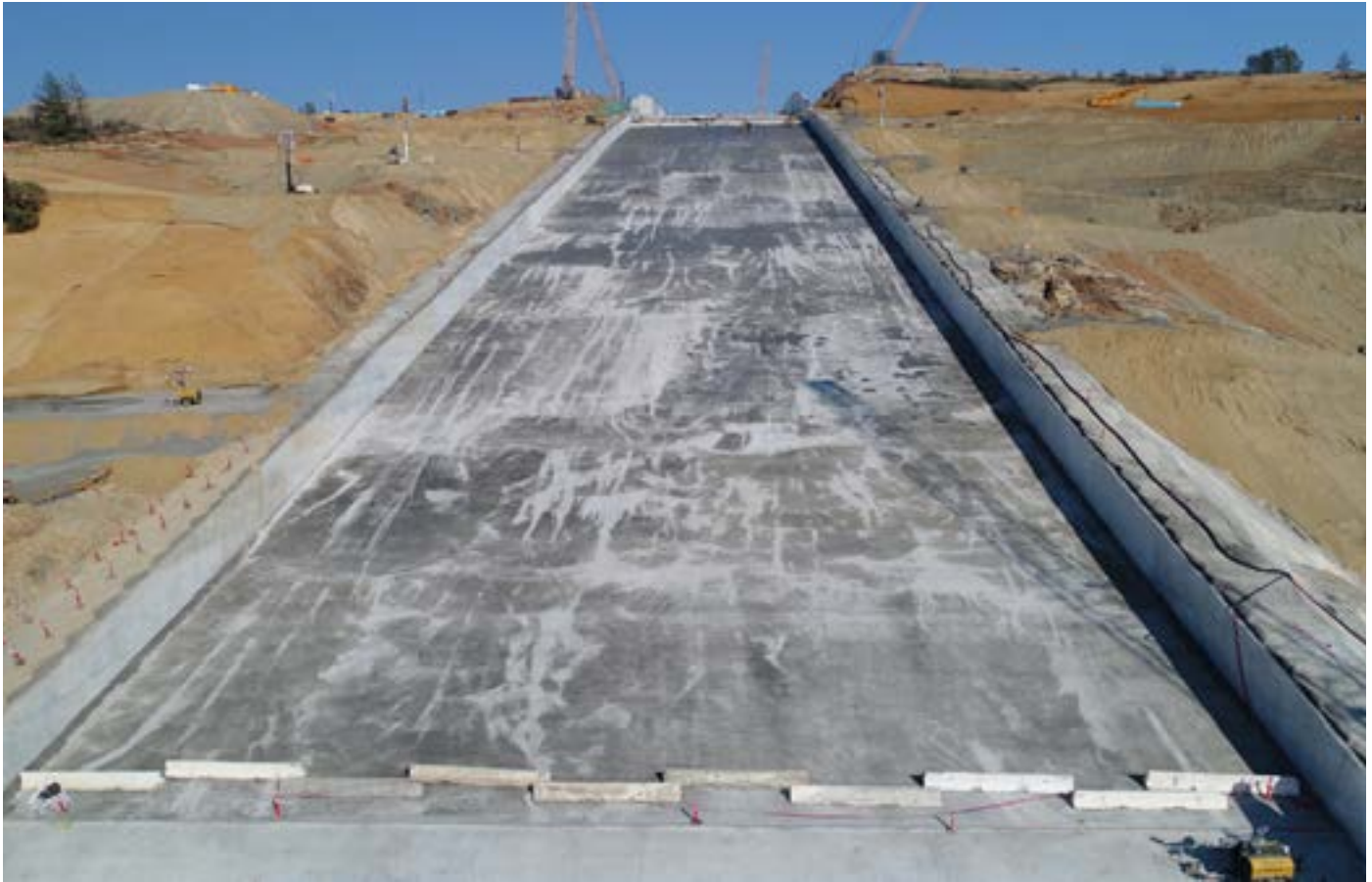
Figure 9. Completed RCC Portion of the FCO Chute (Photo from DWR, November 2017)
