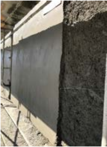
Above: Figure 6. Hilfiker Basket Forming of Vertical RCC Chute Walls
