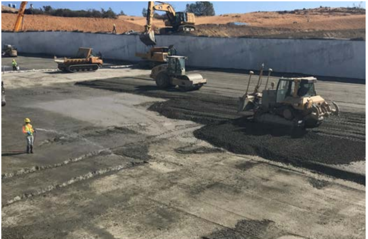
Figure 8. Final Placement of Enriched RCC on Steep 4:1 Chute Slope
