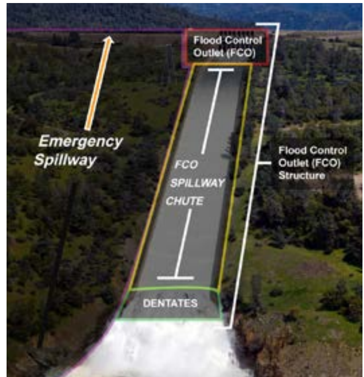
Figure 1. Flood Control Outlet Structure and Emergency Spillway
