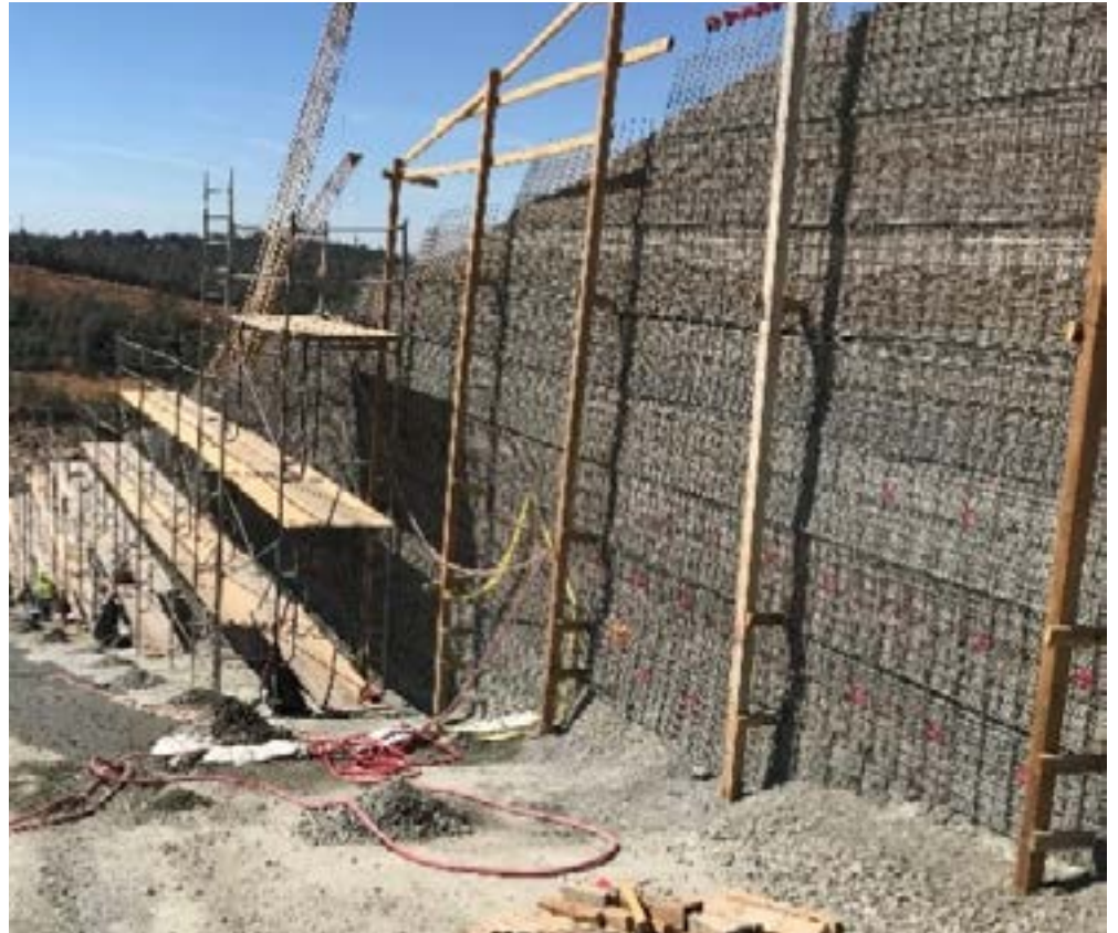
Right: Figure 7. Shotcrete at Inside of Hilfiker Walls
