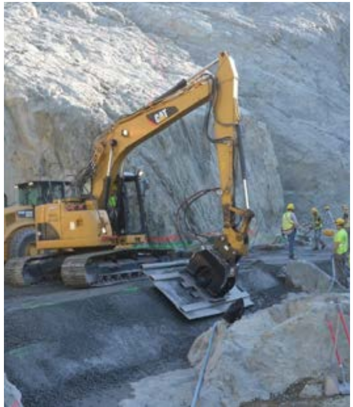
Figure 3. RCC Side Slopes formed at 1:1
